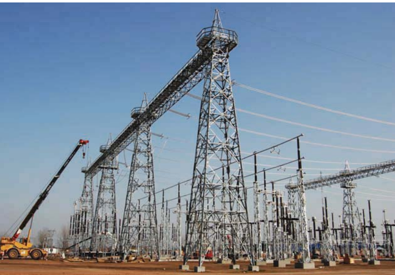
Playa de 500 KW. Será la tercera Central Nuclear argentina. 500 KW yard. It will be the third Argentine Nuclear Power Plant.
