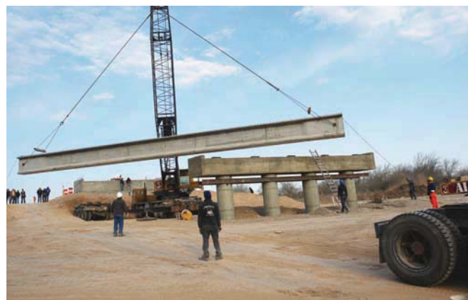
Lifting beams. Bridge over Tortugas Stream.
