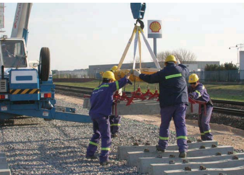
Railways. Placement of mono-block pre-stressed concrete railways sleepers.
