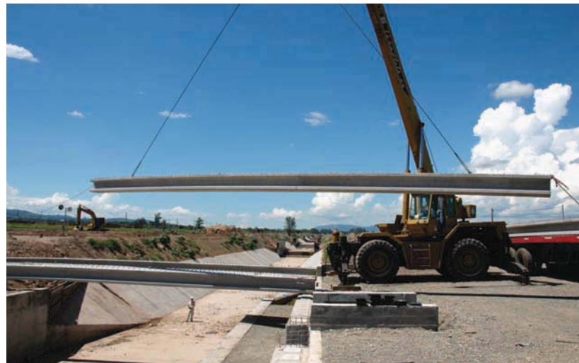
Works. Infrastructure networks and complementary works.
